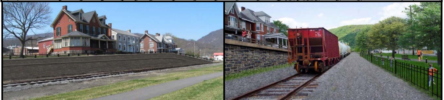
Above , in order: the failing retaining wall overgrown with weeds, the new linear park path, the preliminary design of one of two sections of retaining wall, a rendering of the wall, and a rendering of the future corridor.
